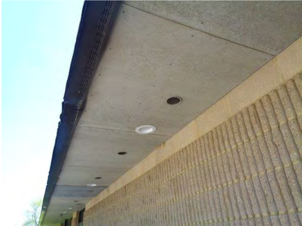
ACM Cementitious Soffit Paneling
