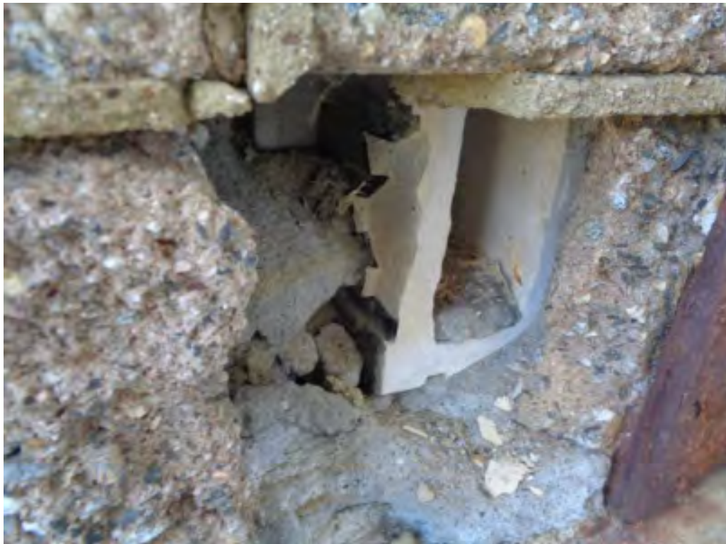
ACM Damp Proofing Behind Masonry Façade and on Terracotta Block
